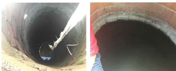
Figure 7. Several wells located in the sliding zone
