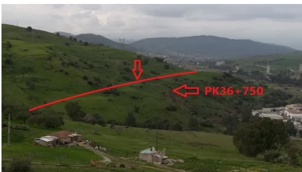
Figure 3. Topography between PK36+600 and PK37+050: View of the foot of the slope, with the sandstone bench
