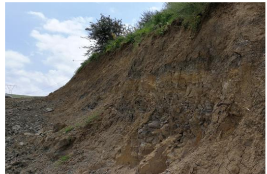
Figure 6. Outcrop of weathered clayey marl
